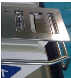
OSB properly maintained
